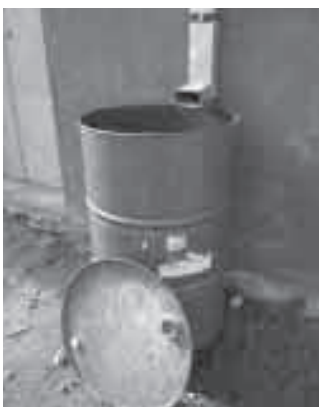
Drum under roof runoff down pipe for rainwater storage within schools.
