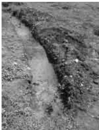
Surface water diversion drain in terraces.
