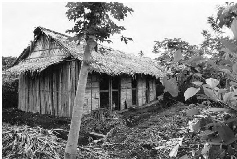
The walls of this kokorako house are made of split bamboo. The roof is made of palm leaf. The garden around the kokorako house produces kokorako food. The ditch around the house drains water away.
