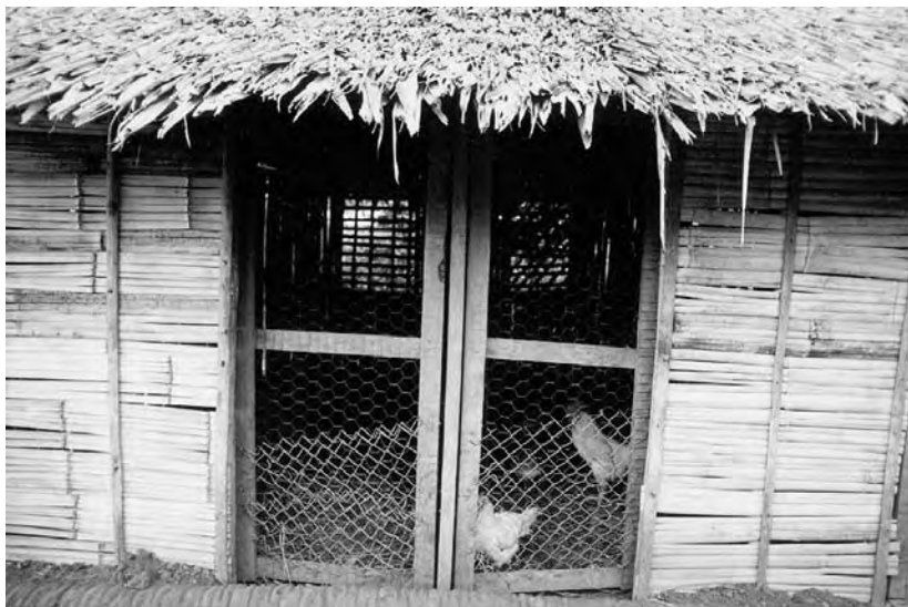
The doors are made of wire mesh on a timber frame.
