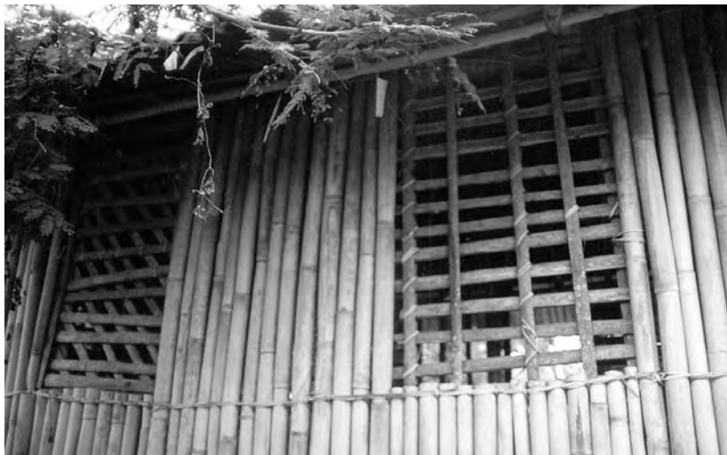
Large windows are provided for ventilation to keep the kokorako healthy and give them fresh air. Smells escape through the windows.
