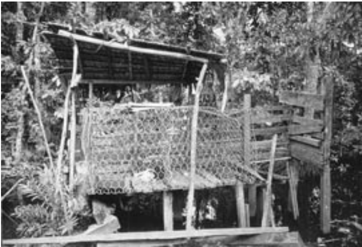
This pig house at Silolo, North Malaita, is built over a swamp. The house has been raised above the water so that it does not flood. Bush poles and cut timber have been used to construct the house. The house provides shelter for two piglets.
